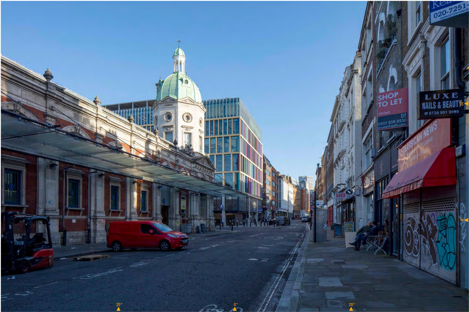
Verified View 05 - Baseline
