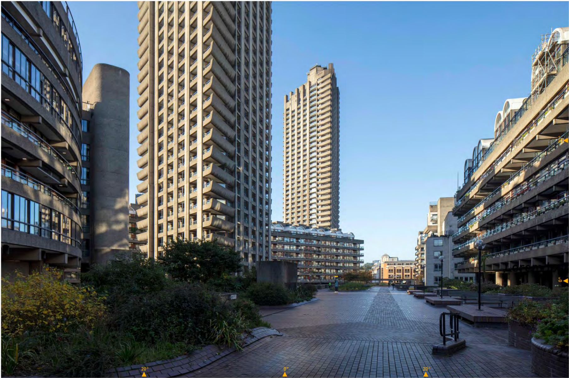
Verified View 09 - Baseline
