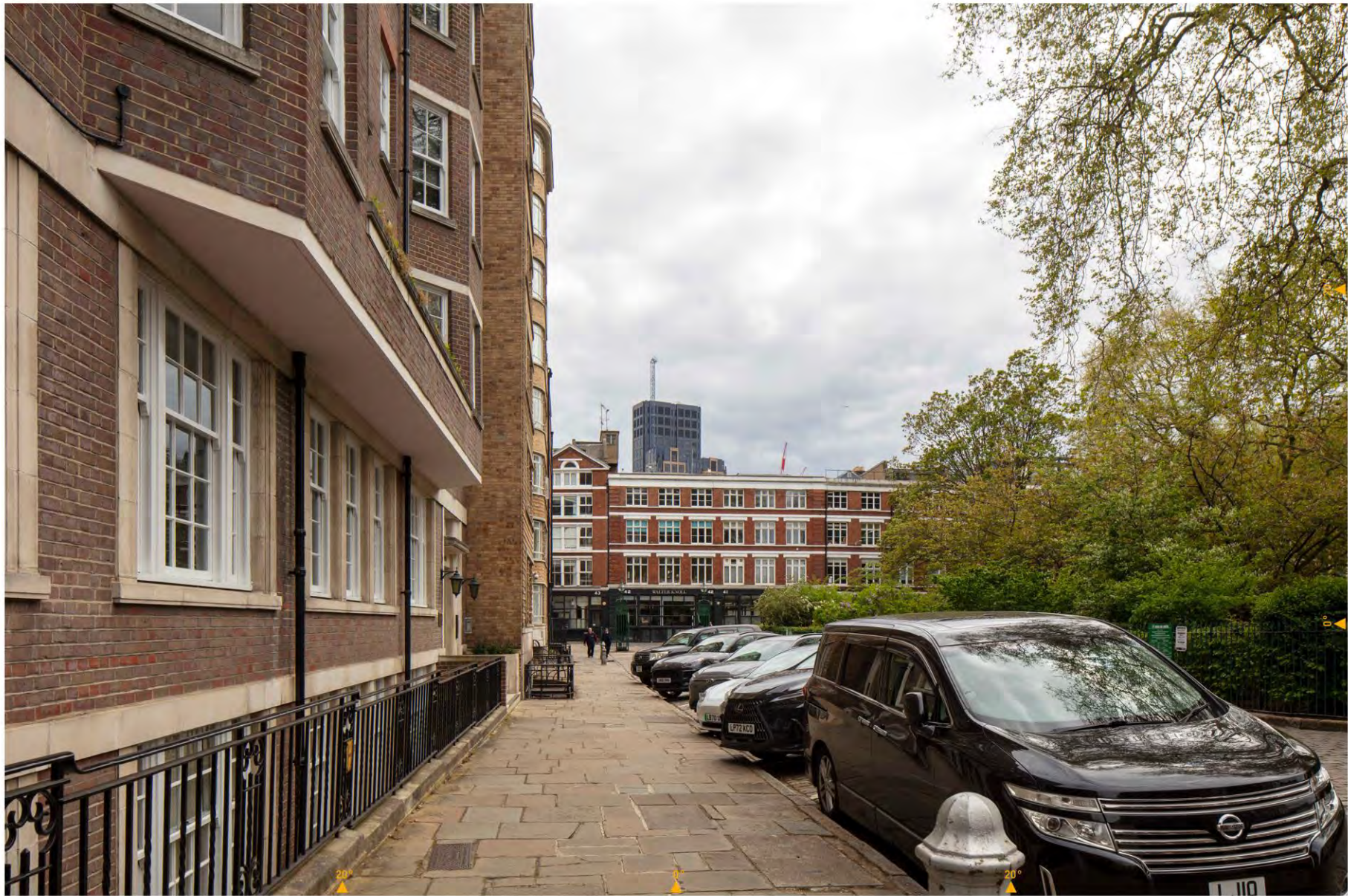
Verified View 12 - Baseline
